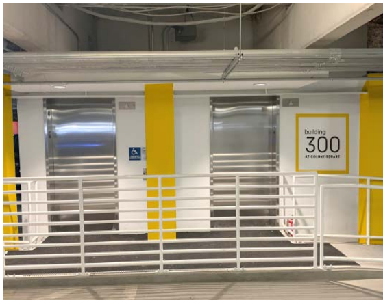
Building 300 Elevator Access. Located on the Red Level.
